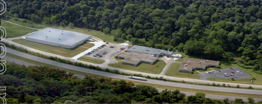
Existing facility located in Triadelphia, West Virginia
