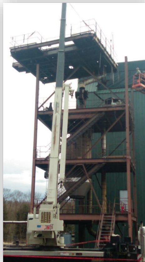
Coal pulveriser system – dismantle operations
